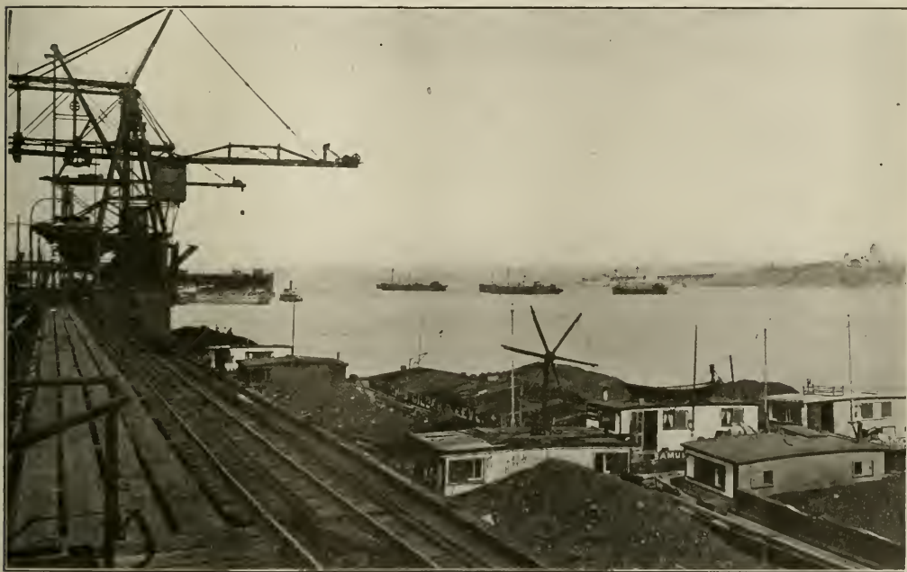
VIEW OF COAL HANDLING APPLIANCE AT SHADY SIDE, N. J.
